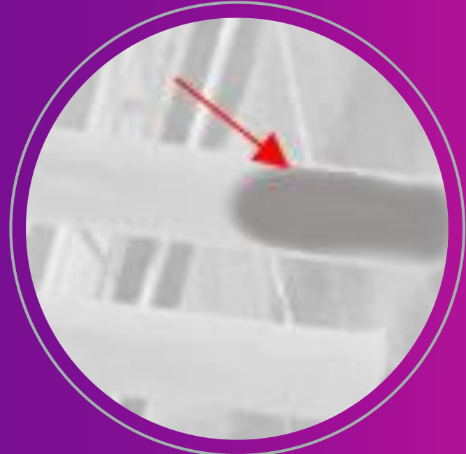
X-ray confirming ice blockage in one of two sprinkler mains
