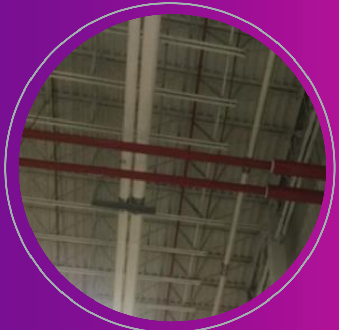
Sprinkler pipes at temperature transition point
